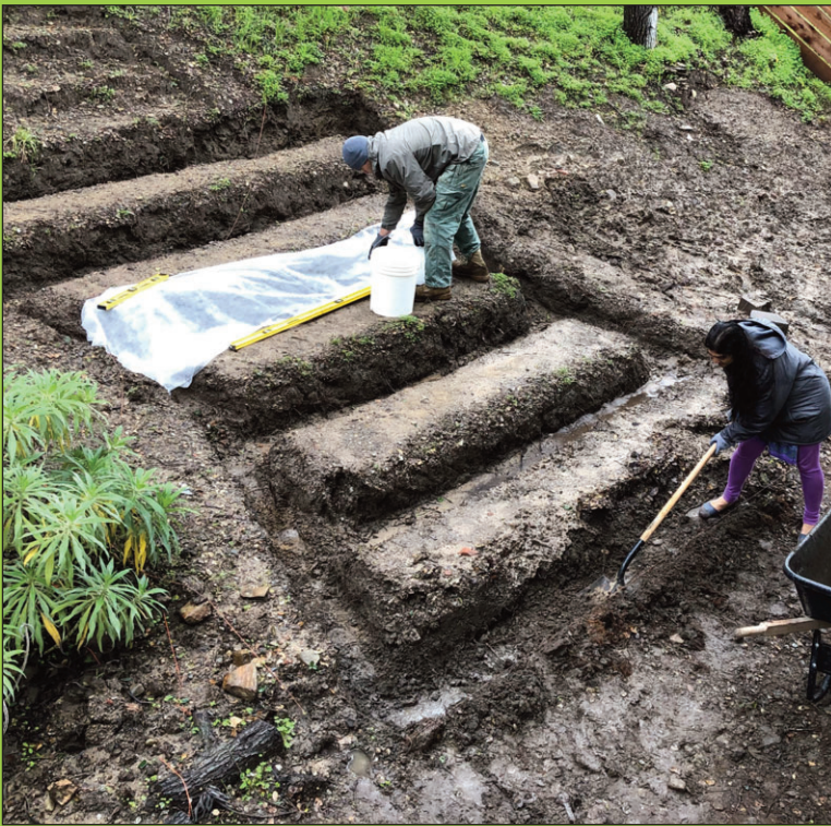
Above: Scott places the plastic tarp upon which the gravel will be poured. Gravel will be used for proper drainage underneath the brick retaining wall.
