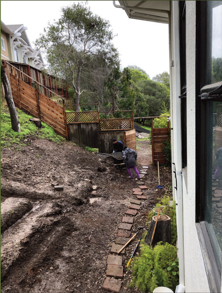
Above: Scott places the plastic tarp upon which the gravel will be poured. Gravel will be used for proper drainage underneath the brick retaining wall.
